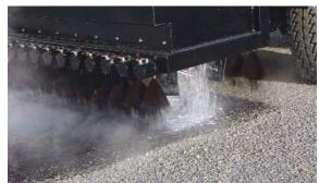
This recognised technique applies of course to the wearing course within the framework of road maintenance by surface dressings. But it also applies in the case of tack coats
