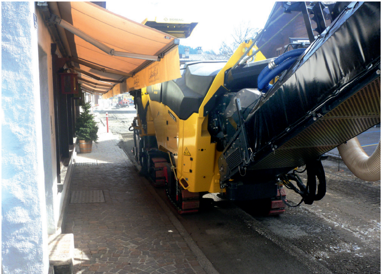
High lateral adjustment and excellent vision from the driver's seat for close-up work near obstacles, saving costly manual rework.
